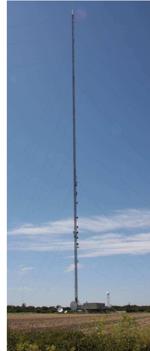
The KCRA Walnut Grove Tower (LBL/CALGEM) equipped with Picarro G1301 CO 2 /CH 4 /H 2 O analyzer with sampling at 30m, 100m and 480m heights.
