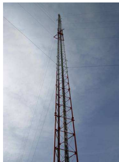
Photos of Penn State tower at Centerville, IA with sampling heights at 30m (100 ft) and 110m (360 ft) above ground level
